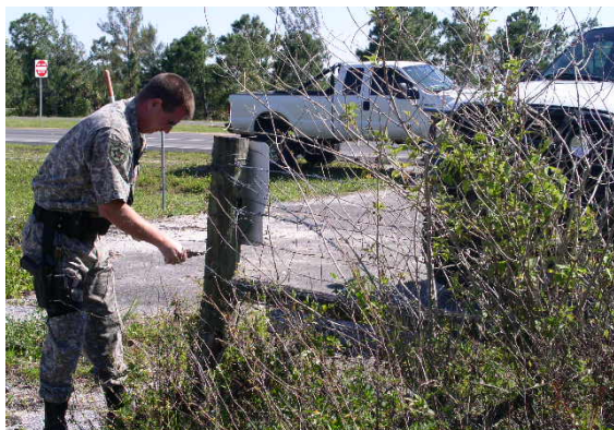
Fence Damage in the Loxahatchee Slough Natural Area
